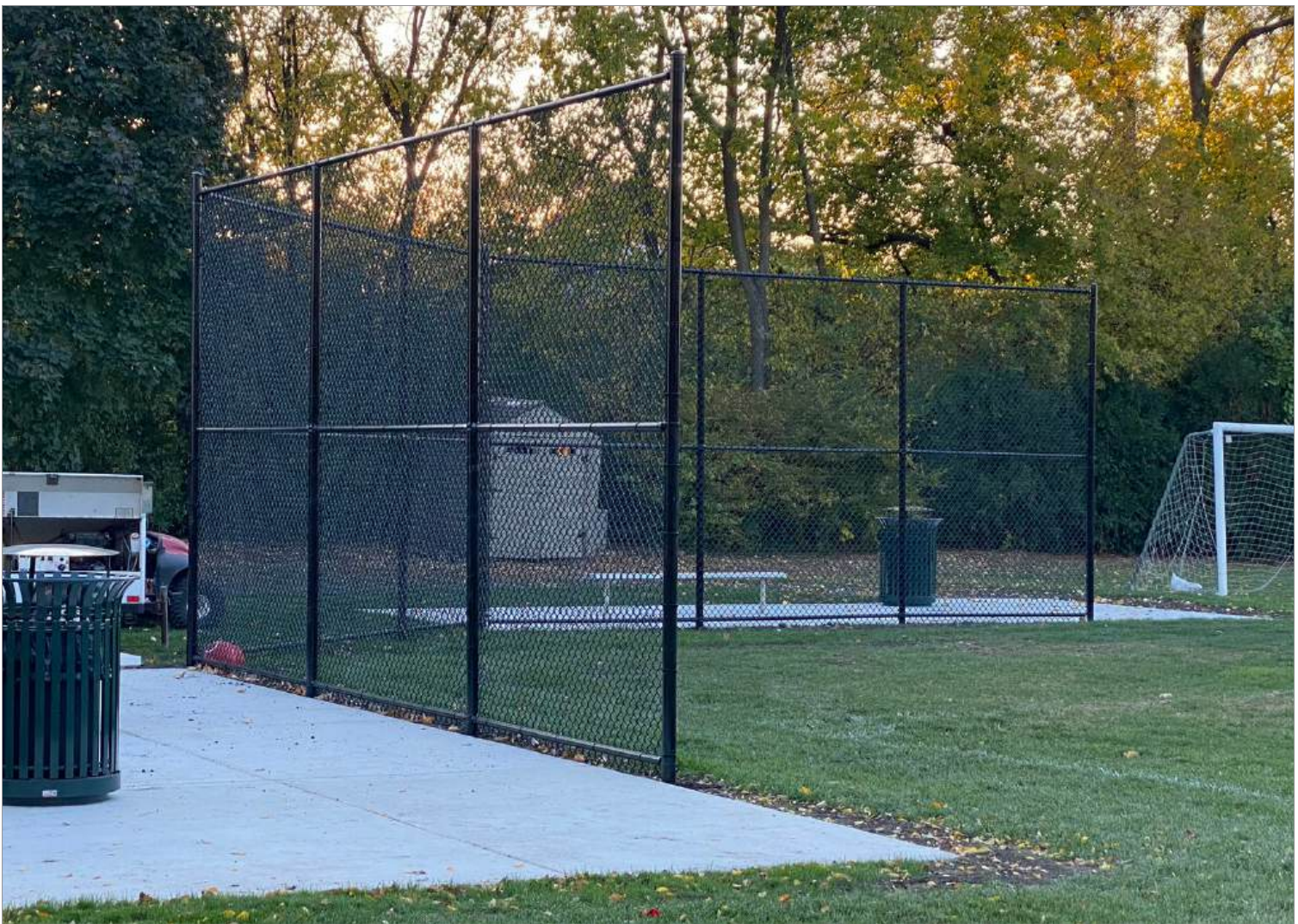
Baseball/softball field renovation with U-8 soccer
