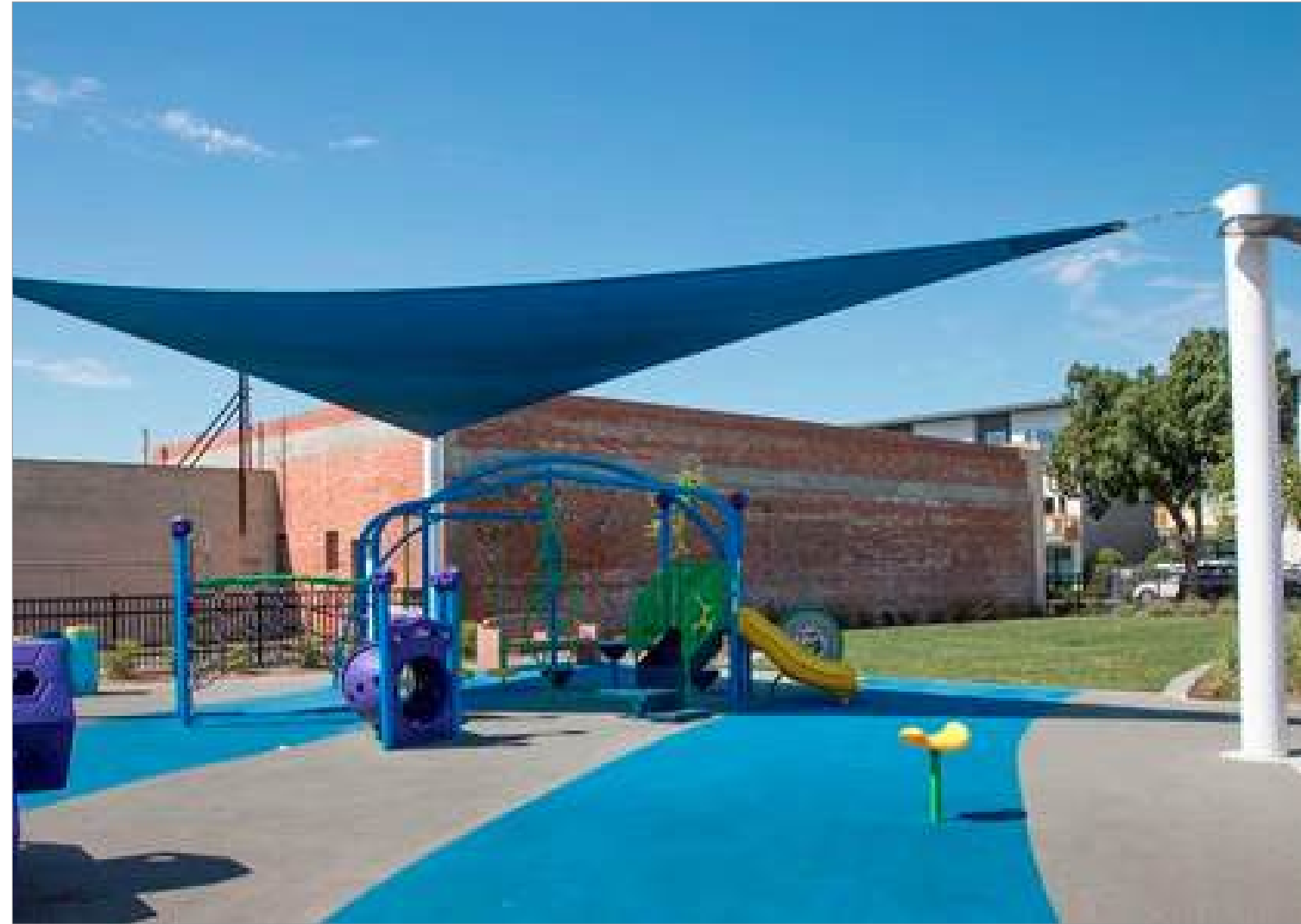
Shade sail structure
