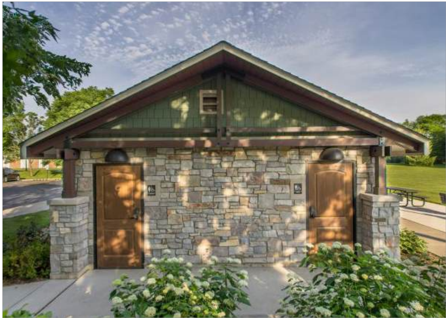
Fieldhouse restroom renovation with outdoor access
