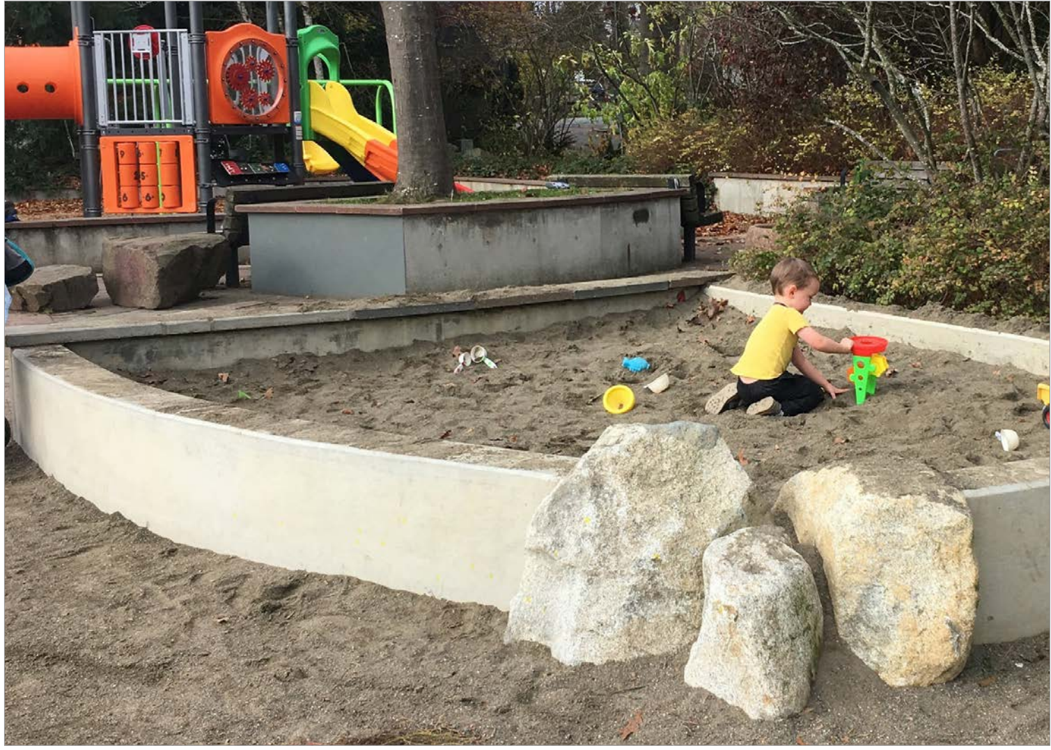
Sand play area with raised concrete seatwall
