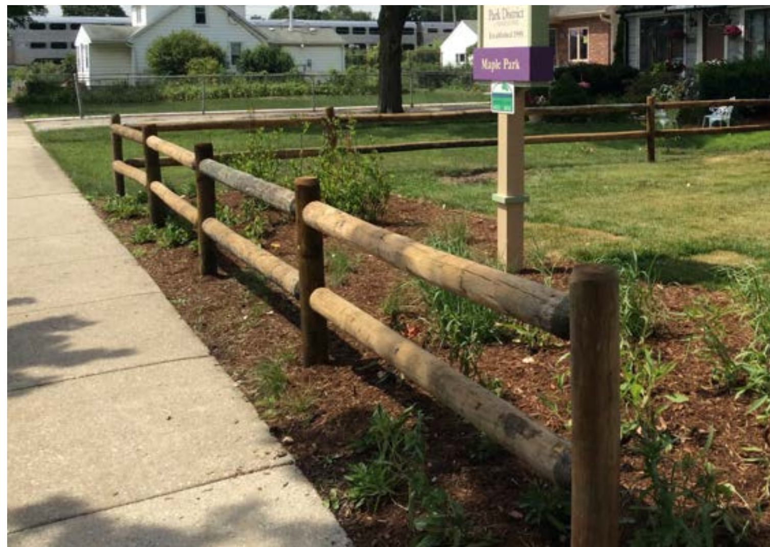
Split-rail wood ornamental fencing
