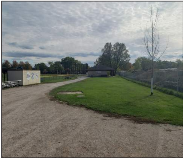
Baseball field 1 / dugout/concession building
