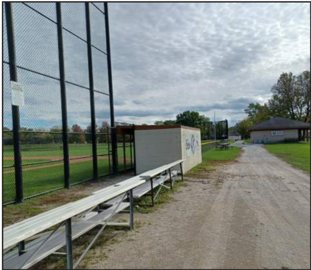
Baseball field 1 / dugout/concession building
